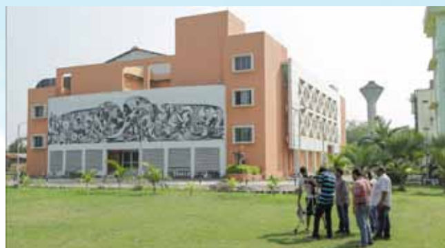
Students at work near newly constructed Film Studio for Television wing at SRFTI, Kolkata.
